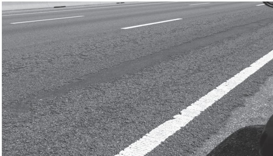
Figure 1. Ravelling in southbound outside lane at Milepost 177.9 (near Prattville)
